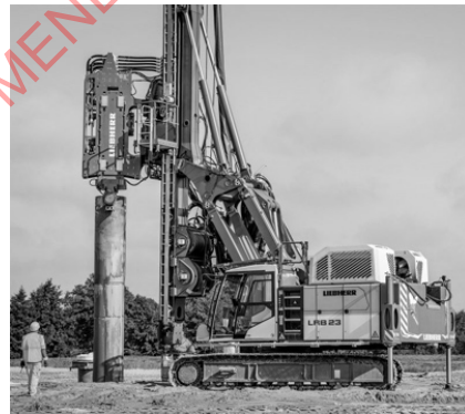
Menanam cerucuk Driving the pile
